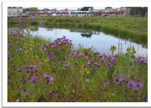
Wet ponds are relatively easy to construct and maintain. Their stormwater management functions include peak rate control and water quality improvement. Photo: rwmwd.org
