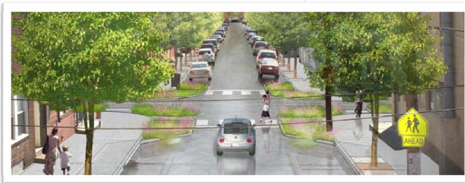
Reducing the impervious area associated with streets and parking can be done through a variety of innovative ways such as installing curb bump-outs (left) or using permeable pavers for parking areas.
