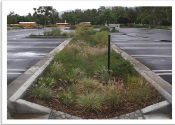
Vegetated swales can be incorporated into a variety of landscapes, including retrofit situations. Above is an example of a parking lot that was retrofitted with a vegetated swale to perform on-site stormwater management and improve aesthetics.
