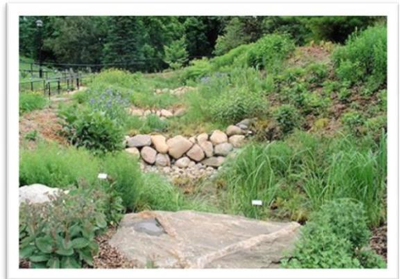
In areas with steep slopes, check dams can be included in the design of a vegetated swale to increase stormwater management performance. The check dams attenuate the water, slowing the peak rate and allowing more time for infiltration.
