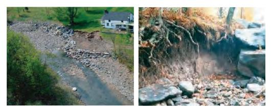
Streambank erosion can occur adjacent to or even behind rock riprap. (Photographs courtesy of Greene County Soil and Water Conservation District.)
