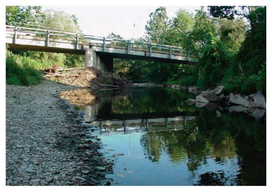
Some bridges are not properly aligned with the stream due to original design miscalculations and/or subsequent migration of the stream. If a bridge opening or culvert is not aligned to the centerline of the stream, the stream's energy will be directed at the embankment, increasing the risk of erosion and consequent damage to the bridge or culvert. (*Photograph of Steuben County Bridge over Meads Creek by Janet Thigpen, Southern Tier Central Regional Planning and Development Board.*)
