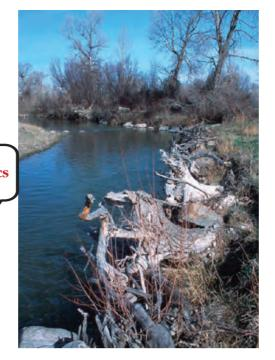
Trees have been buried and anchored in the streambank so that the root wads provide erosion protection. (Photograph by Gary Kramer, USDA Natural Resources Conservation Service.)
