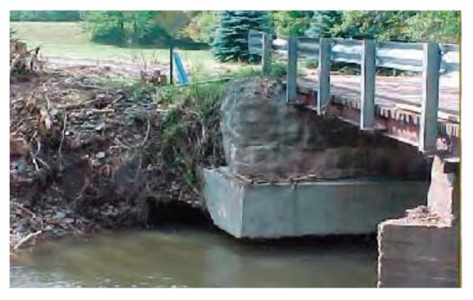
This scour under a bridge is a good visual indication of stream down cutting or degradation. (*Photograph courtesy of Greene County Soil and Water Conservation District.*)
