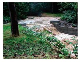
Check dams are a common way of controlling stream grade. A check dam is a structure placed across the stream to control the upstream bed elevation. Steel sheet pile, rock or concrete check dams extending below the level of the bed are used to arrest (check) headcutting. If a check dam is built to extend above the bed of a stream carrying significant bedload, it will trap sediment and build up the streambed to the top of the dam. Check dams can be extremely
