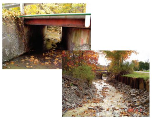
A narrow bridge or culvert restricts the stream channel and blocks flow on the floodplain. Improperly sized stream crossing structures can be a disaster waiting to happen and a money hole for maintenance. *(Photographs by Mark Watts, Chemung County Soil and Water Conservation District.)*
