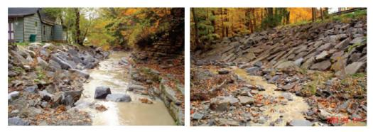
Rock riprap is probably the most familiar of all streambank protection methods and can be an effective means of protecting streamside development. *(Photographs by Mark Watts, Chemung County Soil and Water Conservation District.)*
