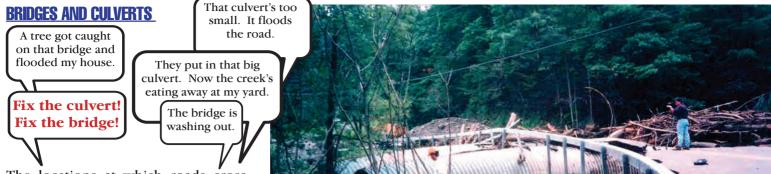
The locations at which roads cross streams seem to be particularly prone to stream problems. This is because the act of constructing a bridge over a stream or channeling stream flow through a culvert almost always alters the stream in a way that disturbs its equilibrium. Some bridges constrict the flow of the stream. Others are prone to accumulating debris, which can block flow. Common symptoms are erosion or sediment deposition or both.
