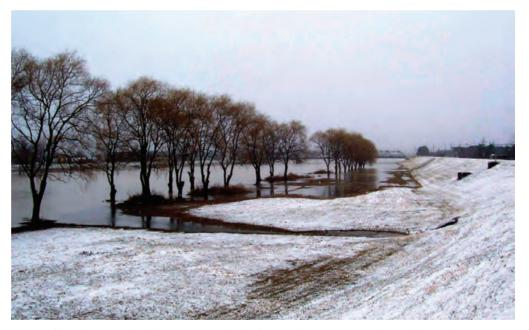
Some flood control dikes are set back from the stream. This allows the stream to function naturally while still protecting nearby land from flooding. Setback dikes maintain a portion of a natural floodplain and provide a floodway where high velocity water can spread out and slow down. *(Photograph by Scott Rodabaugh, NYS Department of Environmental Conservation.)*
