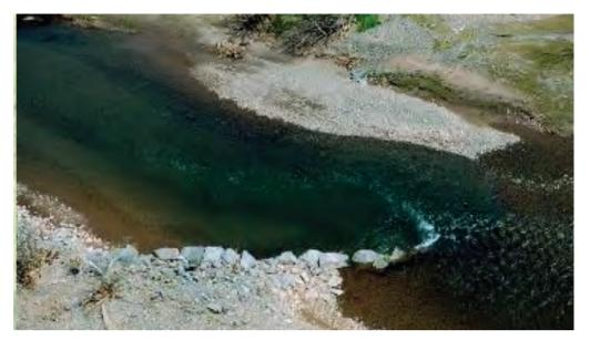
Rock vanes are carefully placed rock structures built below the water level to control the direction of flow within a stream. This vane reduced the velocity adjacent to the streambank, resulting in sediment deposition near the bank on the upstream side of the structure. Vegetation can be planted on this newly deposited material to provide additional protection. *(Photograph courtesy of Greene County Soil and Water Conservation District.)*
