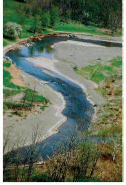
The shape and location of this channel were reconstructed using natural stream design techniques and instream rock structures. (Photograph courtesy of Greene County Soil and Water Conservation District.)
