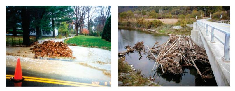
Debris can threaten any bridge or culvert, but if a bridge pier or multiple culvert design splits the stream flow, the risk of debris damage is increased. (*Photographs by Gary M. Patelunas, Town of Elmira Stormwater Department and Scott Rodabaugh, NYS Department of Environmental Conservation.*)
