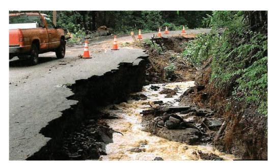
Even in areas that are primarily rural, the increased runoff that results from construction of a few houses, with graded lawns and long driveways, can be enough to wash out roadside ditches and alter stream flow characteristics. *(Photograph courtesy of Town of Campbell Highway Department.)*
