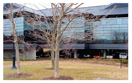
One strategy for floodplain development is to elevate buildings above the height of floodwaters. This protects the new structure and is permitted by most local floodplain development regulations. Although the elevated building may be inaccessible when the surrounding area floods, the building itself is protected from flood damage. The area under this elevated structure is used for parking. *(Photograph courtesy of Steuben County Emergency Management Office.)*
