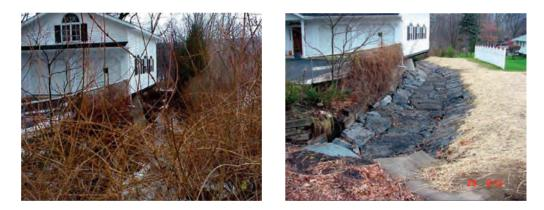
This house was constructed so that a portion of the structure extended over the stream. The builder apparently did not anticipate that the stream would erode its channel ten feet deep and undermine the building foundation (left photo). In order to protect the house, the creek bed was raised, lined with rock, and stabilized with a drop structure – at a cost of \$36,000 (right photo). *(Photographs by Gary M. Patelunas, Town of Elmira Stormwater Department.)*
