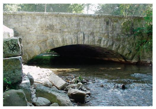
Aggradation of the stream has significantly reduced the capacity of this bridge, which now causes flooding of surrounding areas. *(Photograph courtesy of Herkimer-Oneida Counties Comprehensive Planning Program.)*
