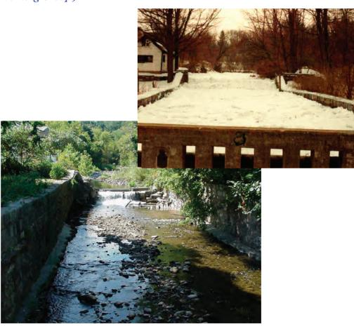
This channel was designed to carry a stream safely through a residential neighborhood. Unfortunately, the narrow channel and a low bridge clearance restrict the flow of ice, causing ice jams at this location. *(Photographs courtesy of Herkimer-Oneida Counties Comprehensive Planning Program.)*
