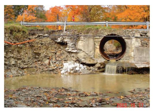
Water shooting out of this culvert has blown out the banks of the downstream channel. (*Photograph by Mark Watts, Chemung County Soil and Water Conservation District.*)
