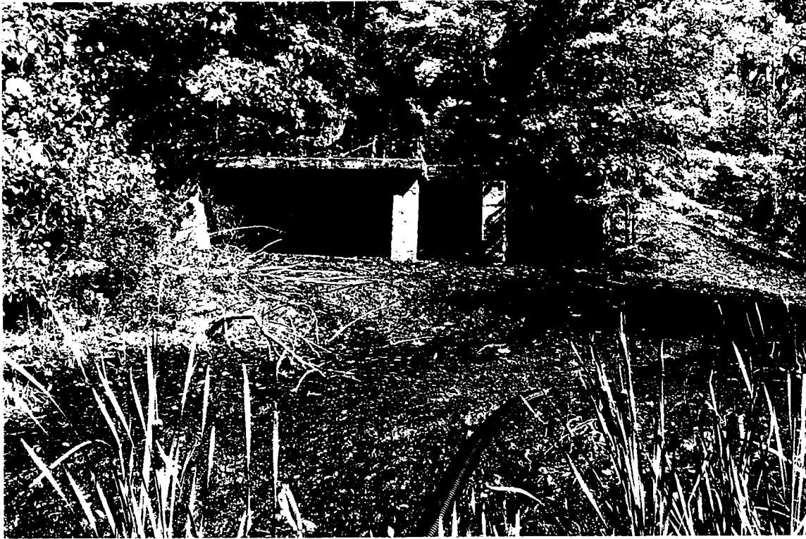
Site 8 originates at this mine opening located just downstream of site 7 along SR2011. The discharge flows through a culvert under SR2011 and continues into Dunkard Creek as shown in the photo below.
