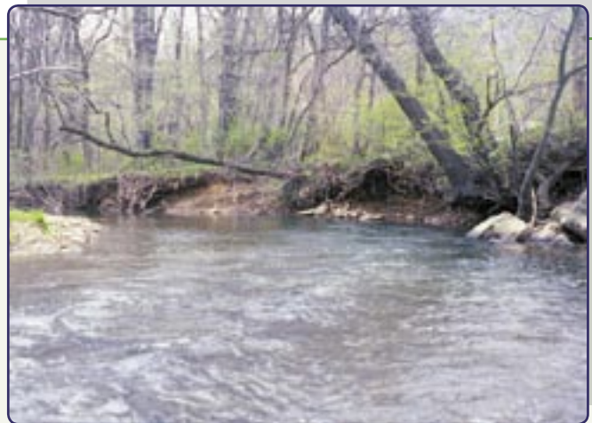
Bank erosion in the Mallard Lane area.
