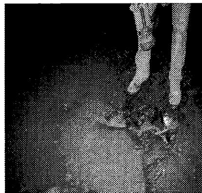
Holes have been identified within 100 yds of the Braddock Avenue culvert (a culverted tributary). This significantly affects stream flow and may be adding to SSO and chronic discharge loading of sanitary sewers.
