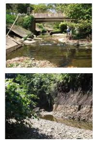
Even the most sturdy bank armoring designs have proven unequal to the force of West little Pine in its southern reaches. Here, a road is in jeopardy if the wall fails.
