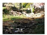
A deteriorated railroad tie retaining wall is no longer serving its original purpose and could contribute flooding debris to create dams in a storm event.
