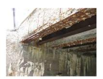
The decaying infrastructure of bridges such as this one on MP3 impacts stream quality and increases the risk of the structure failing in a high flow event.
