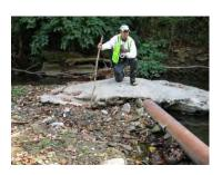
Erosion also threatens utility infrastructure. Here a pipe that had originally been cemented over is now exposed.
