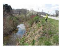
MP3 along McKnight Road has several pipes that are at severe risk of collapse as the streambank has eroded away, leaving them suspended and without support.
