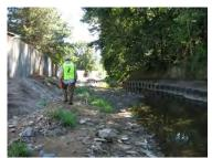
The lower reaches of West Little Pine have received large volumes of sediment from the upper portions of the watershed during storm events. In some areas the deposits have become problematic because they reduce the capacity of the constricted channel during high flow events.
