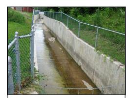
Jack's Run, a subwatershed of Sewickley Creek, is enclosed within concrete channels in multiple sections throughout its drainage.
