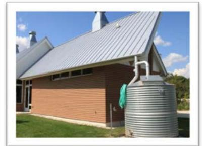
Some of the variations of runoff capture and reuse include underground storage (above left), rain barrels (above middle), and cisterns (above right). These systems are often implemented with other BMPs such as vegetated swales, rain gardens, and/or pervious pavement to maximize stormwater management performance.
