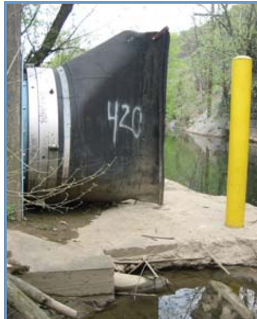
Combined sewer discharge structure located in Pine Creek, Pa.
