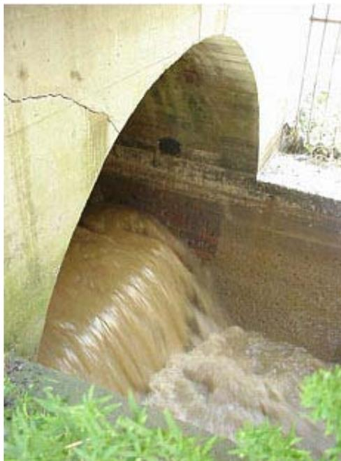
**Photo 11. Combined Sewer Overflow.**
