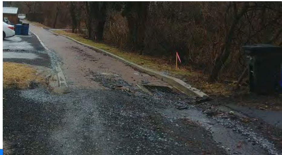
Figure 3-3. Baffles on Steep Slope Baffles used in a sloping permeable pavement application increase the storage efficiency (Source: EPA Green Infrastructure Technical Assistance Program Addressing Green Infrastructure Design Challenges in the Pittsburgh Region: Steep Slopes, January 2014)
