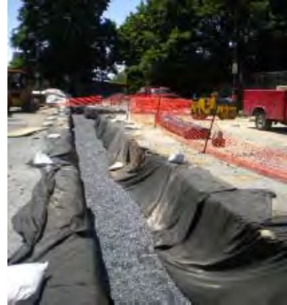
Left side: correctly installed geotextile Right side: incorrectly installed geotextile
