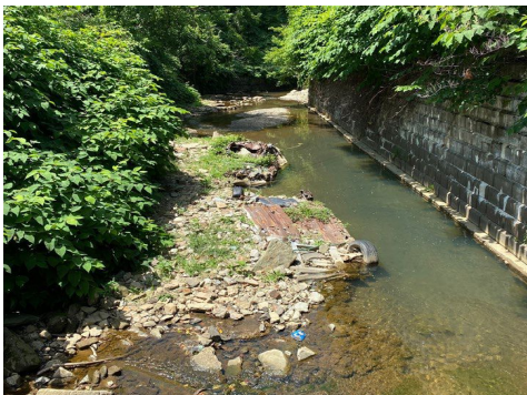
Typology 4 Vertical streambanks or walls/private land
